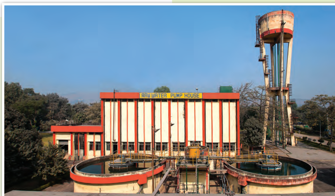
Raw Water Pump House at Rourkela
